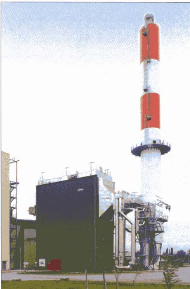
SCR-Reactor after Electrostatic Precipitator
