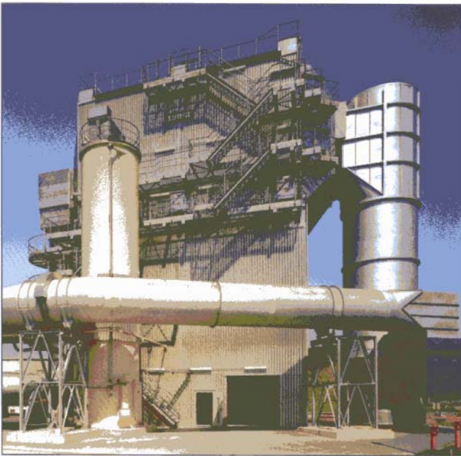
Reactor with dry additiv and Electrostatic Precipitator
